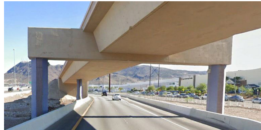
Figure 3.13 Existing I-515 SB On-ramp Bridge
