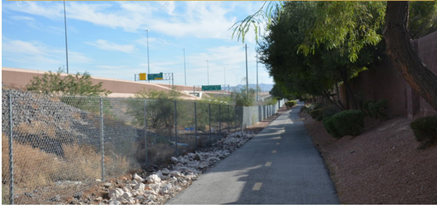
Figure 3.12 Key Viewpoint 1 – Existing Condition – I-215 south side looking northeast towards South Gibson Road Interchange
