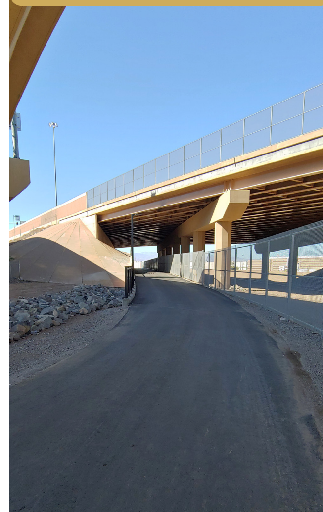
Figure 3.26 UPRR Trail Looking North
