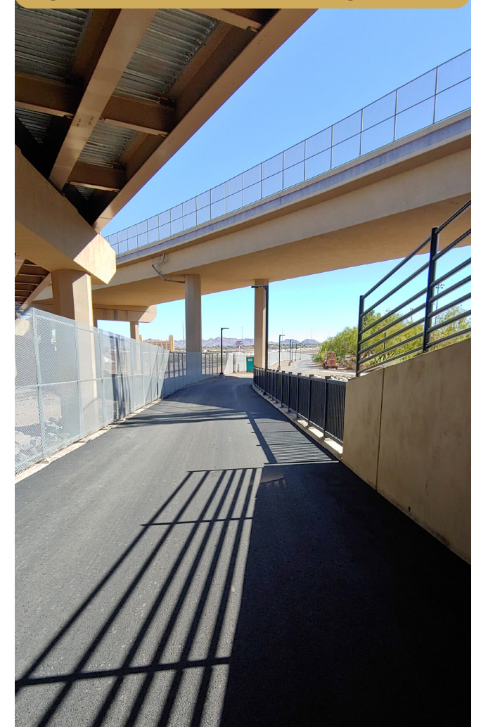
Figure 3.27 UPRR Trail Looking South
