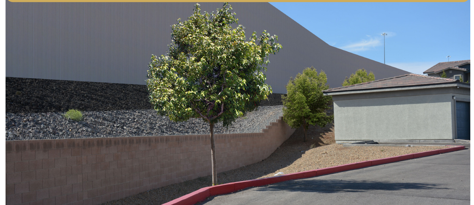
Figure 3.21 Key Viewpoint 5 – Build Alternative – View looking west to the I-215 from residential neighbors in multi-family homes at the Dream Apartments from Wigwam Parkway west of Gibson Road where units are on the north side of I-215
